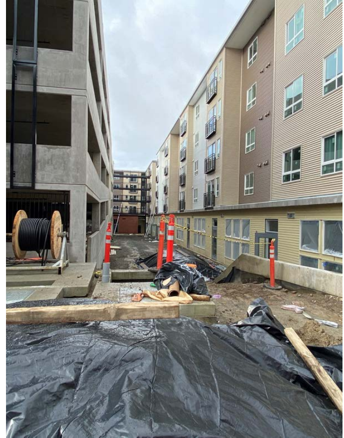
North internal courtyard – Live/Work Units
